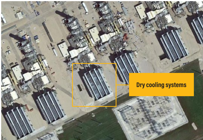
Figure 7 | Satellite Image of a Dry Cooling System
