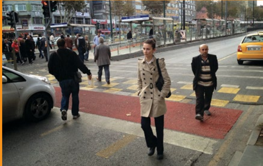
A raised crossing in Istanbul helps give priority to pedestrians at an access point to a tram station.
