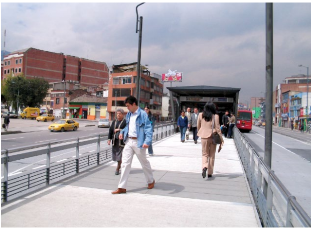
Figure 54 TransMilenio 2006: A pathway between two substops at the same station. Note the low guardrails, approximately 1 meter in height. Because they were so low, people could jump over them easily, and this was a major pedestrian safety risk.
