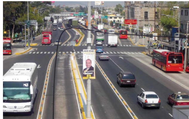
Figure 86 Eje 3 Oriente after intervention, showing BRT lanes for Metrobús Line 5 and improved pedestrian infrastructure
