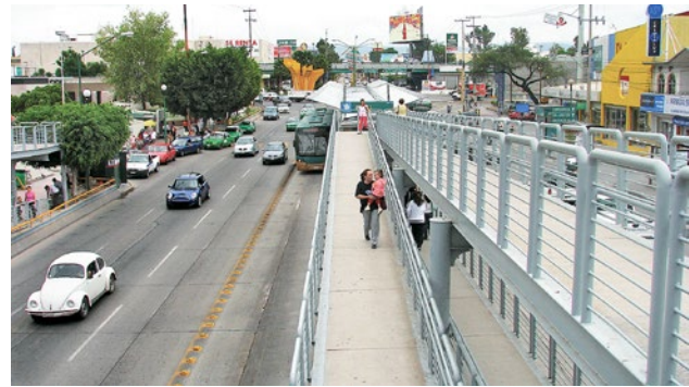
Figure 13 Pedestrian bridge with ramp and resting area in León, Mexico
