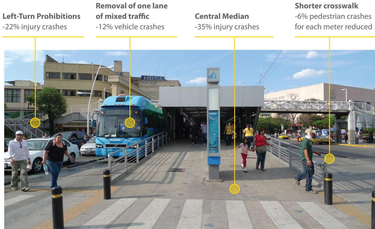
Figure 2 Changes to the street infrastructure to accommodate a typical Latin American BRT (here, Macrobus, Guadalajara) and their associated safety benefits
