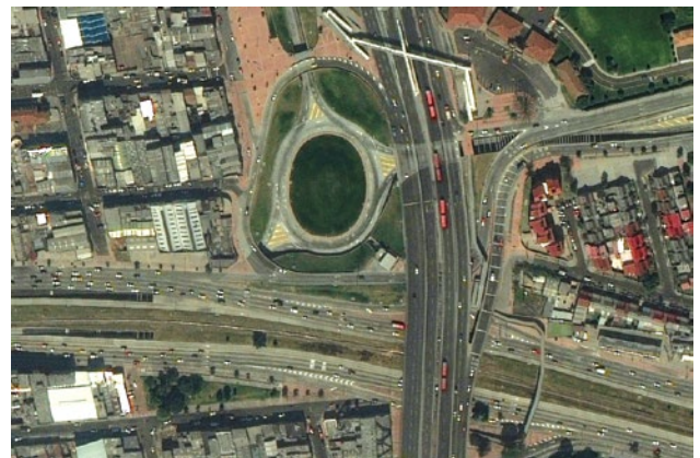
Figure 74 Junction between three TransMilenio corridors: NQS, Calle 80, and Avenida Suba. Bus connections between the three corridors are done via overpasses and underpasses, which maximizes capacity for all the movements and minimizes potential conflicts between buses.
