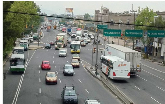
Figure 85 Eje 3 Oriente Eduardo Molina before intervention, showing counterflow configuration and a switch in driving direction
