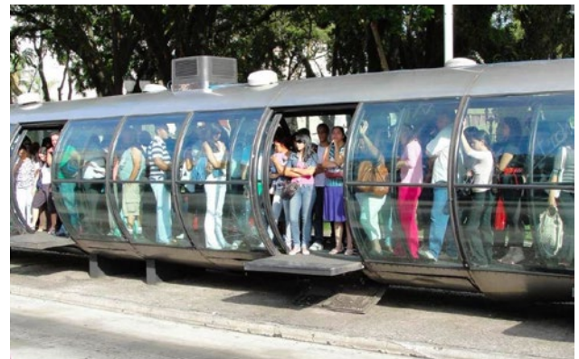
Figure 53 A platform screen on a BRT station in Curitiba. The doors are open, even though no bus is present. This is a safety risk in a crowded station, as passengers can accidentally fall into the bus lanes.
