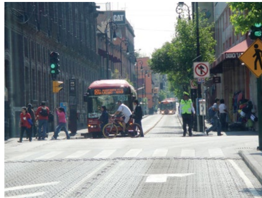
Figure 46 New traffic signs and pavement markings indicating the end of a shared lane and the beginning of a dedicated bus lane, where mixed traffic must turn right
