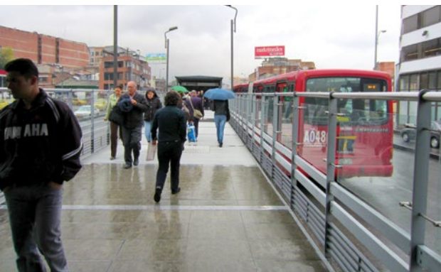
Figure 55 TransMilenio 2011: The guardrails along the pathways were raised to make it more difficult to climb over. We recommend using this higher type of guardrail on any pathway connecting different parts of the same station
