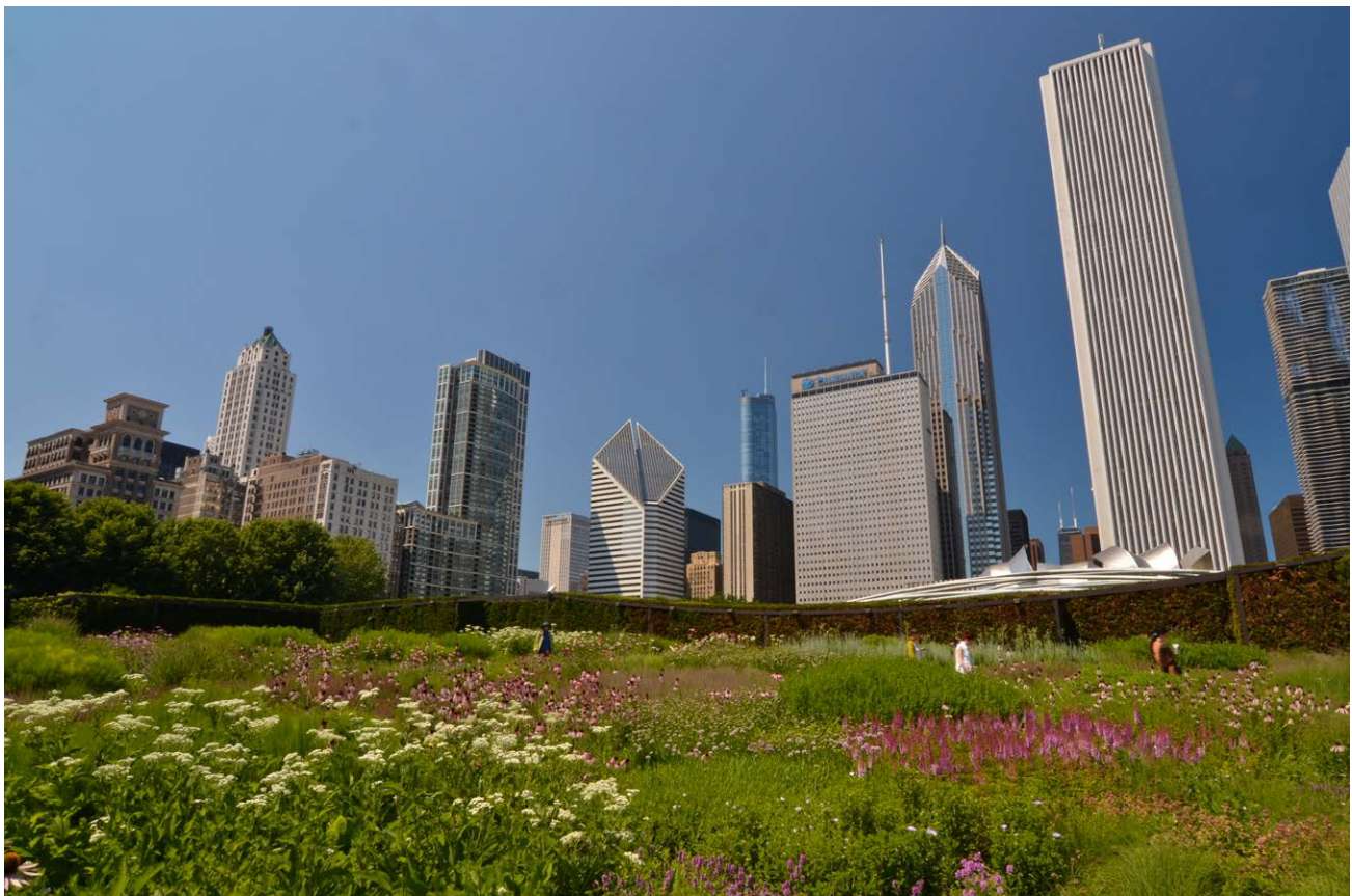
Figure A4 | Green Roof Atop a Parking Garage and Rail Yard in Illinois That Helps Slow Stormwater Runoff
