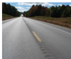
2-Lane Roads 80–90km/h (Milled rumble strips)
