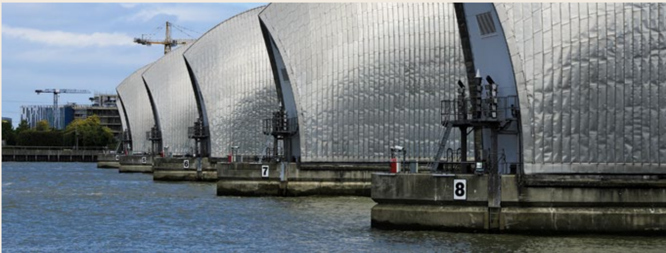
The Thames Barrier works to hold back storm surges and high tides protecting 1.3 million people.
